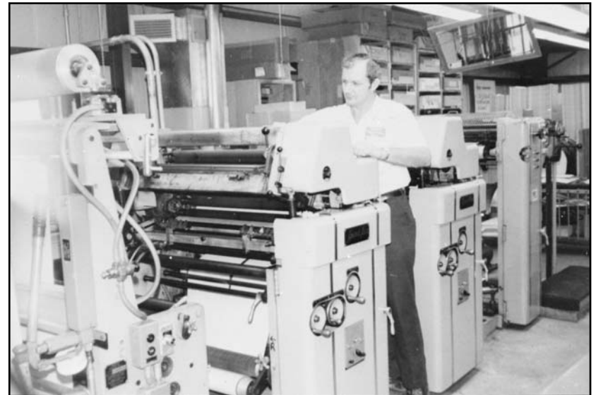
Ott Beer ran the two-unit web press purchased in 1966. This $48,000 press could produce eight times as much printing as the Harris and saved 13 percent on paper costs by using rolls of paper instead of sheets.
